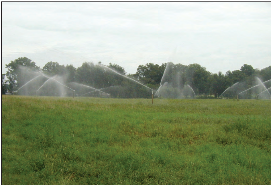
The Inverness Wastewater Treatment Plant Restricted Access Sprayfields— One goal of this project is to end the regular irrigation of these fields just to return the city's wastewater back into the aquifer.
